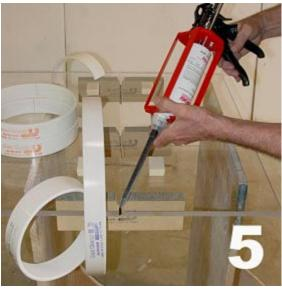
4. Dry fit the deck seam and check for 5. Open the seam 1/4" and apply enough 6. Push the adhesive to get squeeze out on both the top and bottom. No need to overdo it.
